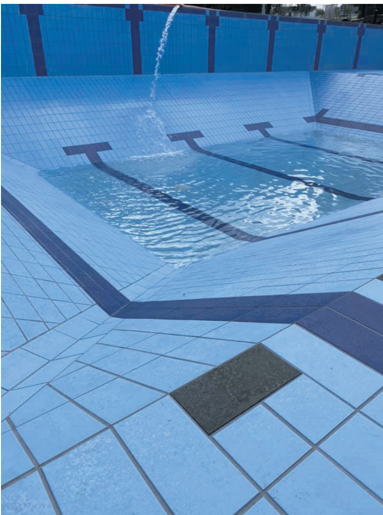
Pool tiles complete and pool filling in process
